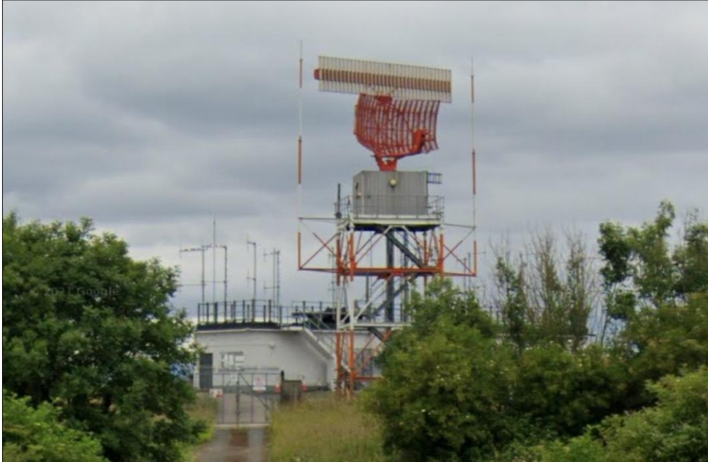
Figure 11. Dublin Airport MSSR Radar Station #1
