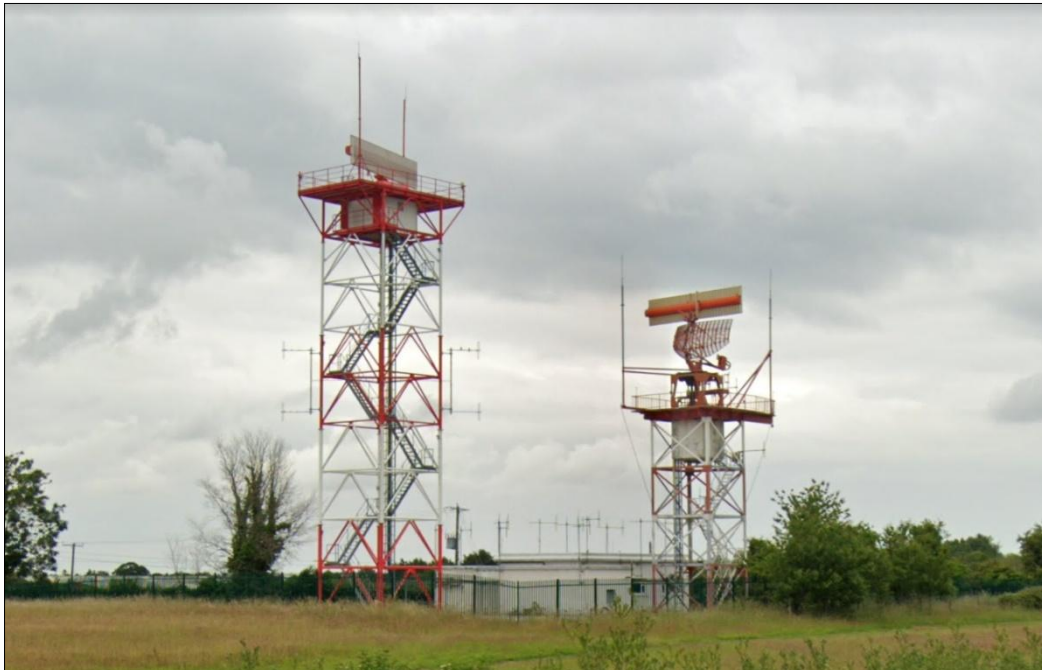
Figure 12. Dublin Airport MSSR Radar Station #2
