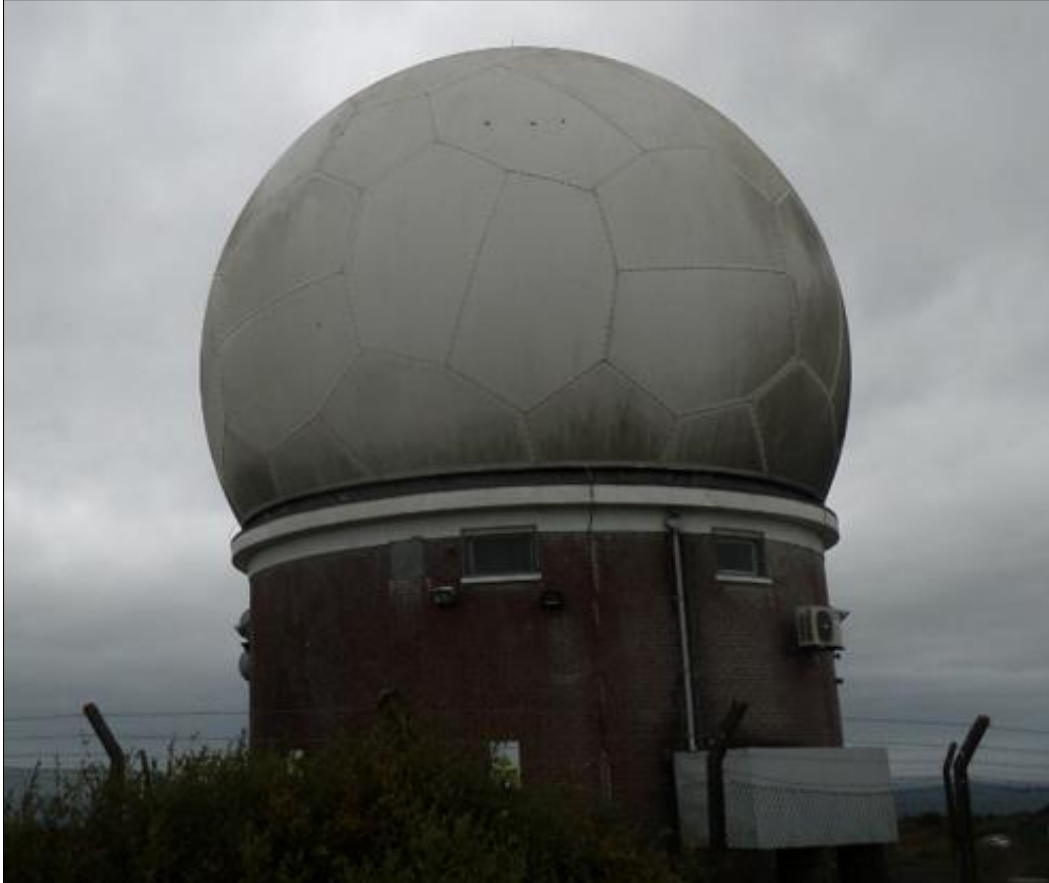
Figure 10. Woodcock Hill Radar Station
